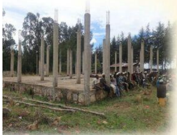
Phase 2 Current Condition 1/2 Million Birr has been spent
